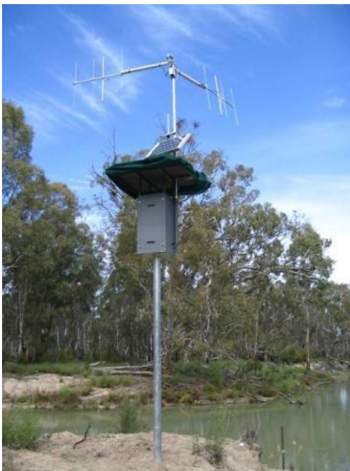
Figure 2. Upper Mullaroo data logger, showing logger box, solar panel and antennae.
