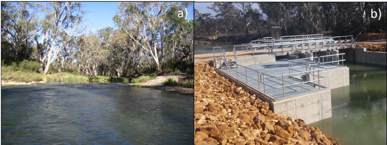
Figure 9: The Upper Mullaroo Creek in a) 2014 with the old ford structure and, b) 2016 with the construction of the new regulator/fishway.
