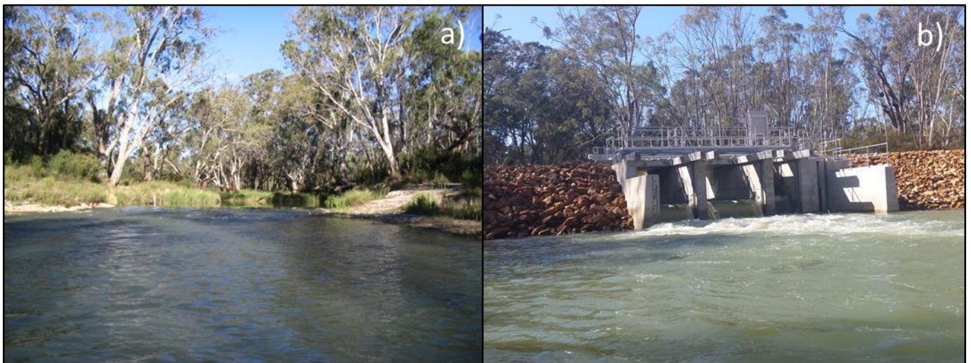
Figure 14. The Upper Mullaroo Creek in a) 2014 with the old ford structure and, b) 2016 with the construction of the new regulator/fishway.
