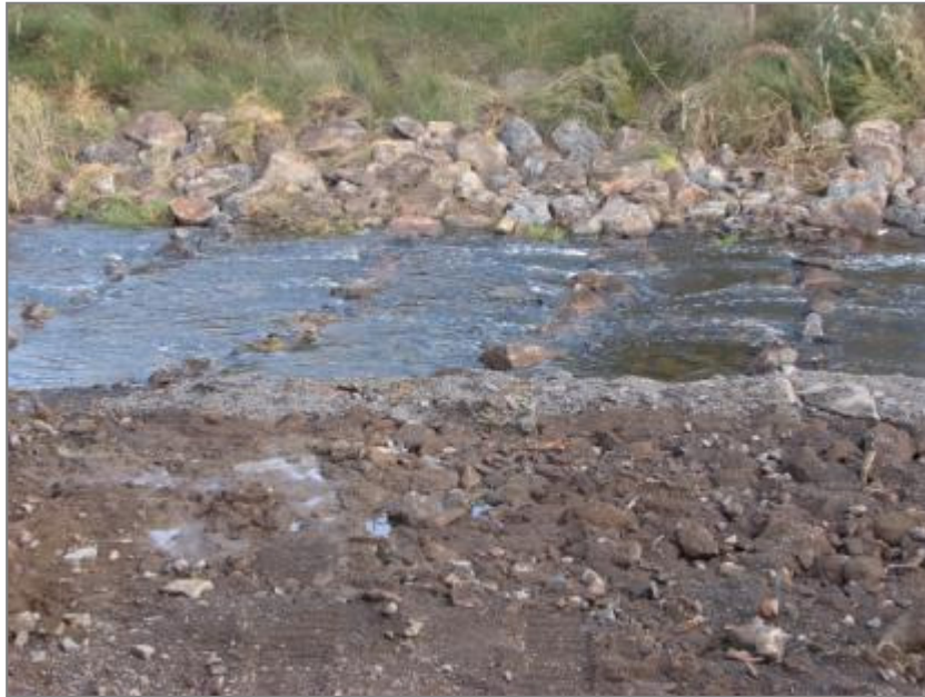
Figure 16. A well-designed lateral ridge rock fishway with large pools and small drops for fish to ascend a weir. These design features could be incorporated into the Thompson's Weir rock fishway. Commissioning the fishway by making small adjustments to the rocks over the design flow range was an important aspect in achieving an excellent fishway.
