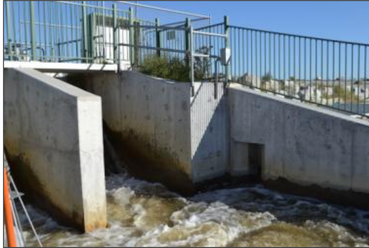
Figure 14. Entrance of Gunbower Weir fishway (31/3/2011) subject to high turbulence from Gate 1 spill flow (209 ML/d).
