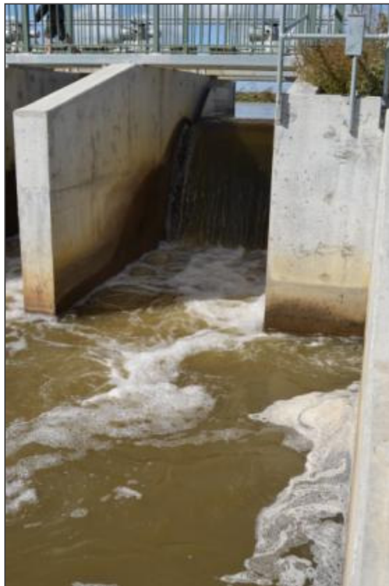
Figure 15. Optimised attraction with a reduced Gate 1 spill of 50 ML/d (23/4/2011).
